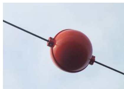
Avian marker spheres are of international orange, gloss white, gloss yellow, and other colours, of which yellow is effective, reflecting light at dawn and dusk, and contrasting with backgrounds better than international orange
