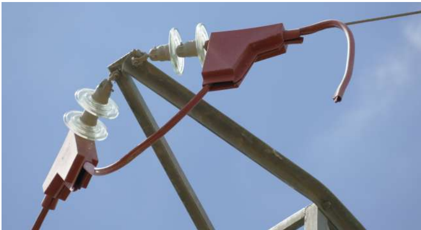
Twisted, insulated conductors reduce collisions by increasing visibility in distribution lines
