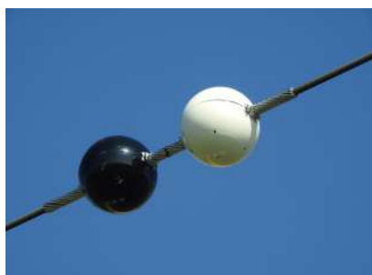
Avian marker spheres are of international orange, gloss white, gloss yellow, and other colours, of which yellow is effective, reflecting light at dawn and dusk, and contrasting with backgrounds better than international orange
