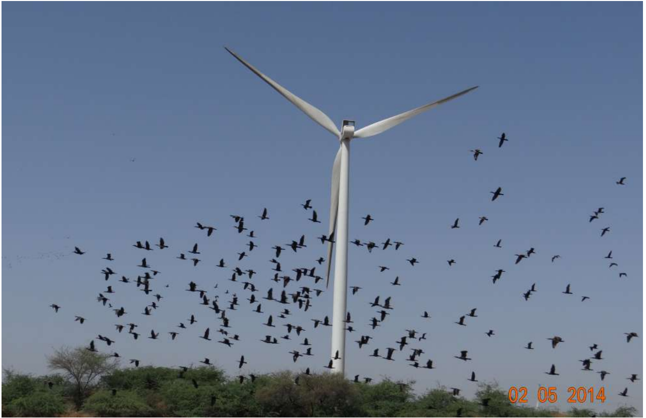
A wind turbine near a wetland in Kutch, Gujarat
