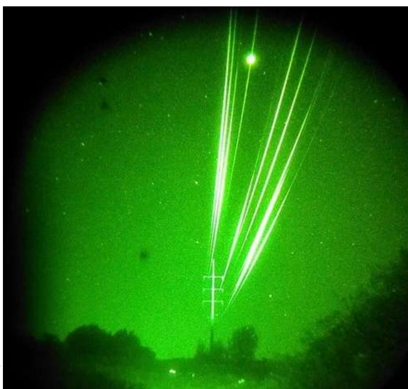
Green laser lights installed on power lines indicated reduction in seabird collisions on Kaua‘i Island, Hawaii, USA
