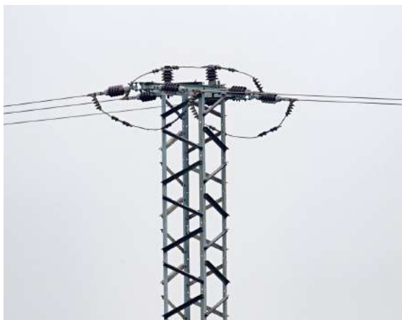
Image 8: Changing the construction of the dangerous pole to more bird-friendly pole
