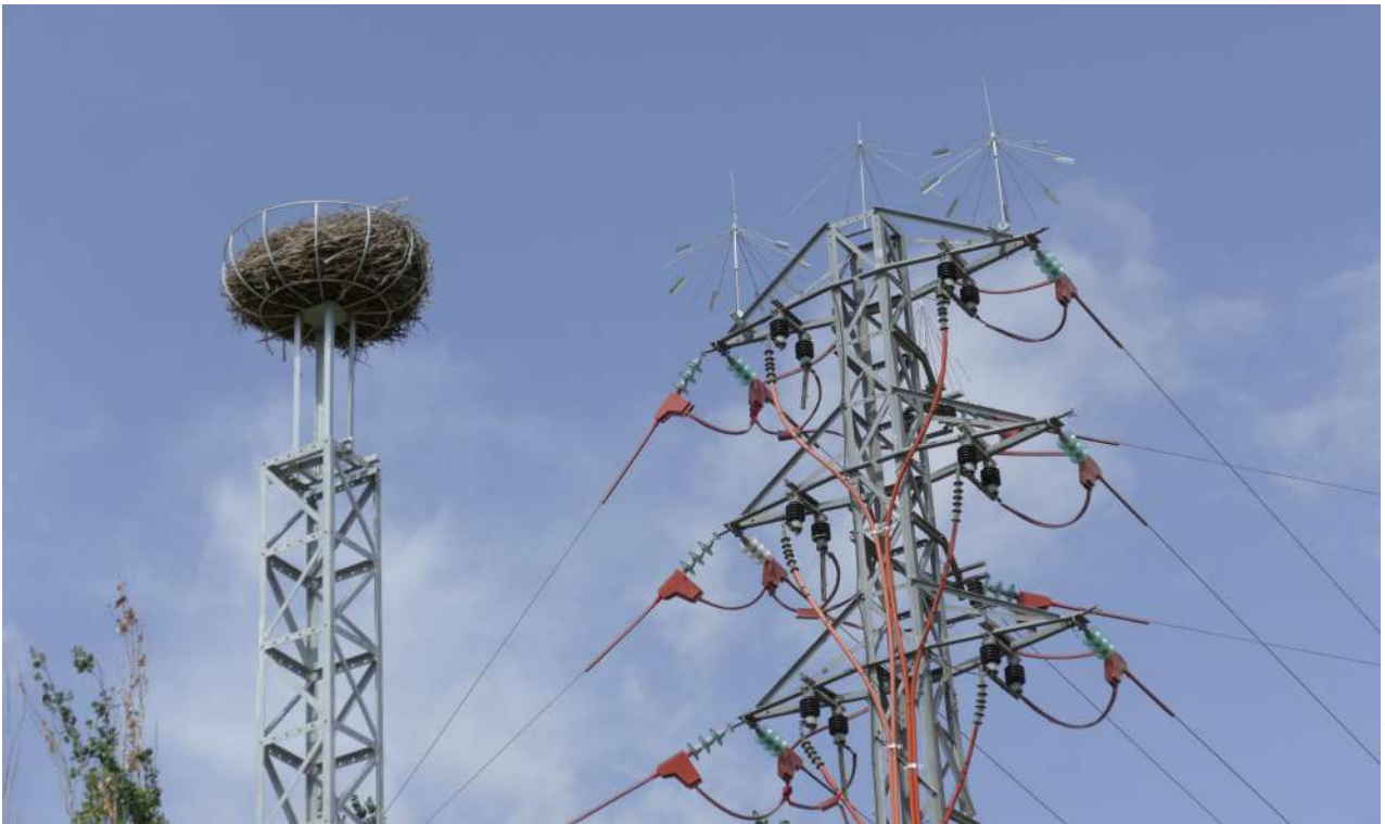
Effective anti-electrocution measures (Top Left): A White Stork Ciconia ciconia perching on a raised structure atop a pylon and an anti-perching deterrent; (Top Right): Raised structure for nesting purposes with a White Stork Ciconia ciconia nest; (Bottom): Utilization of anti-perching deterrents combined with a nearby artificial nest alternative
