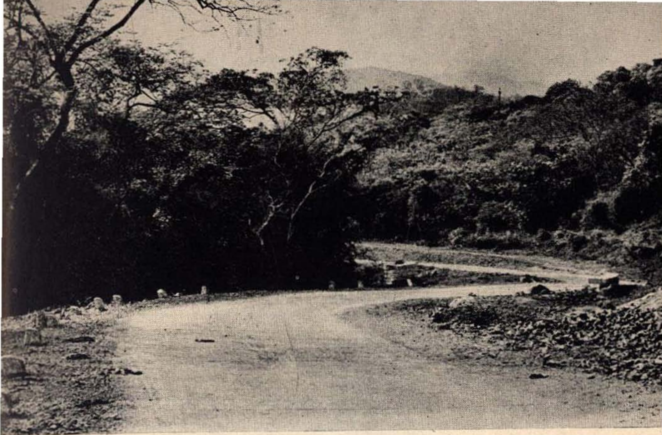
The road through Borivli National Park which was realigned. (Note the clearing on the right of the picture. This is being replanted.)
