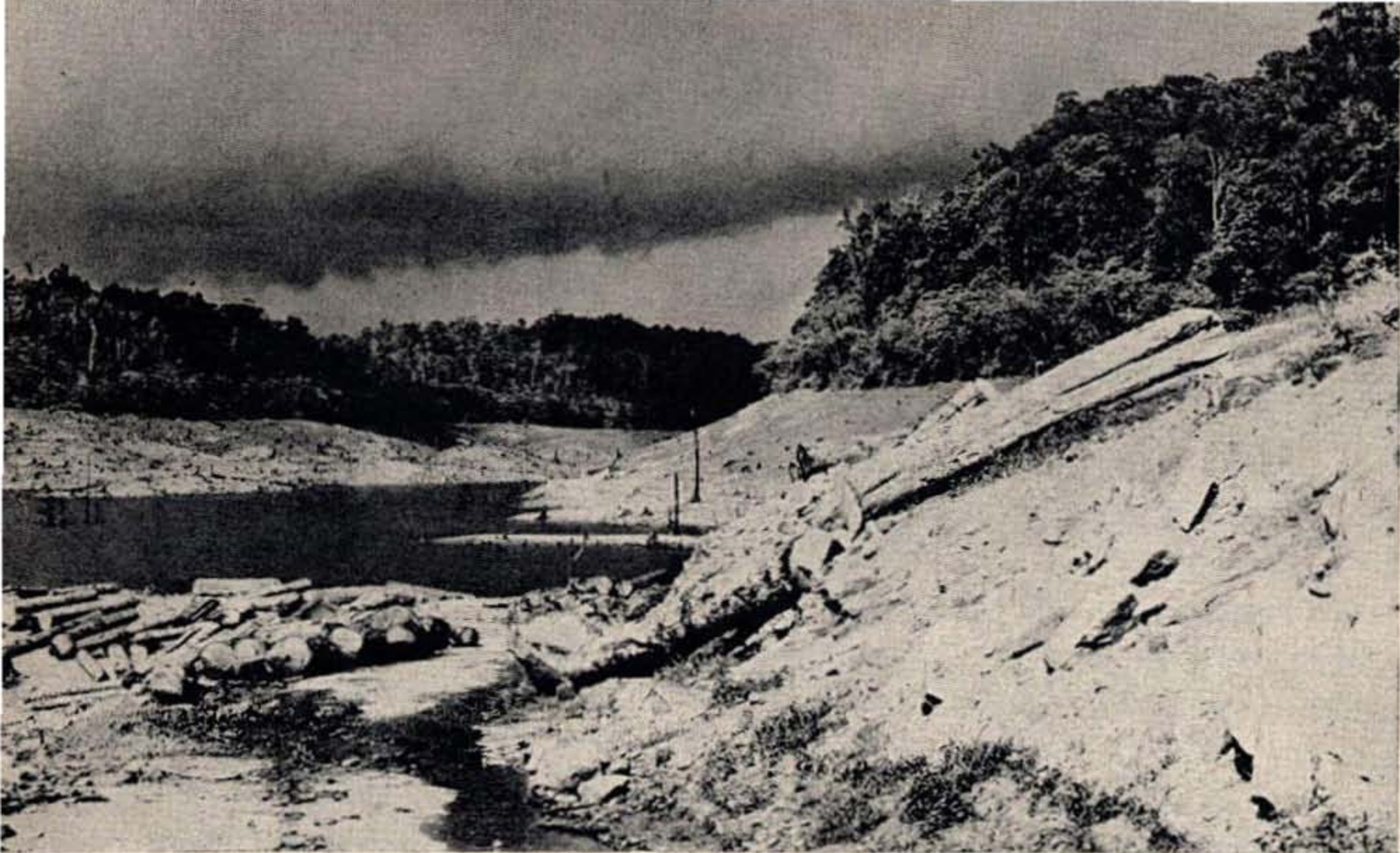
Sholayar Dam Reservoir
