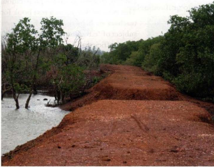
Bunding is done to prevent saltwater intrusion directly affecting the mangroves
