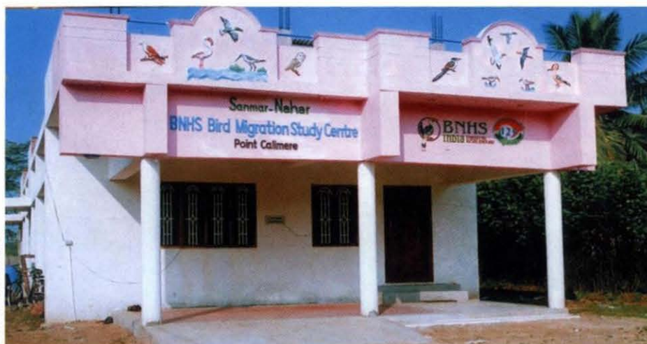
▲ The recently built Bird Migration Study Centre of the BNHS at Point Calimere
