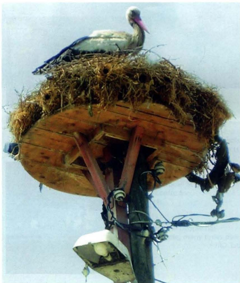
Stork nesting tray secured to electricity pole near Uluabat lake, Turkey
