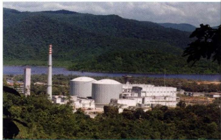
Kaiga Atomic Power Station comprises four units each of 220MWe, of which two are under operation (shown above) and two under advanced stages of construction.
