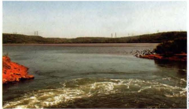
The area affected due to bund
