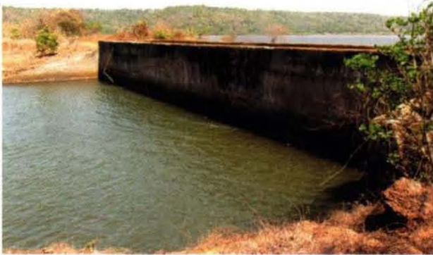
Bund constructed on Jaigad Creek near Kasari
